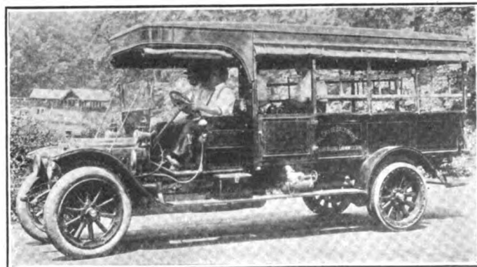
White truck in the service of the Electrical Commission of the City of Baltimore, which, in addition to performing manifold duties, is fitted with a wireless receiving station by means of which it keeps in constant communication with the office
